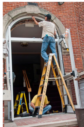
The new front doors and flooring were installed this week.
