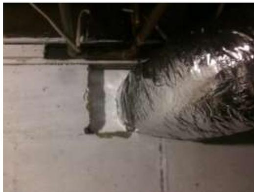
Attic air leaks are also a concern in both the Church and Annex, but are not yet carefully characterized. (Cold air enters the attic area as part of the normal process, but should not be allowed to enter walls or the interior space.) The situation is uncertain at present and may be 5% to 20% of the heating cost, thus warranting further evaluation.
